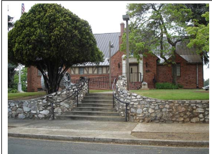
Rock Wall at Veteran's Memorial Hall
